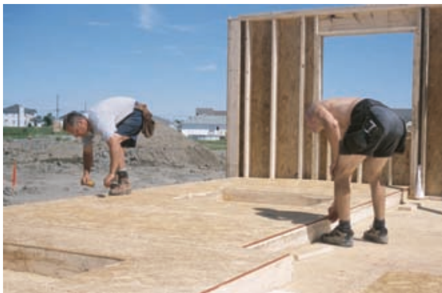
Designers, specifiers and contractors may want to evaluate on a project-specific basis whether moisture-related risks make it appropriate to use OSB or plywood.
